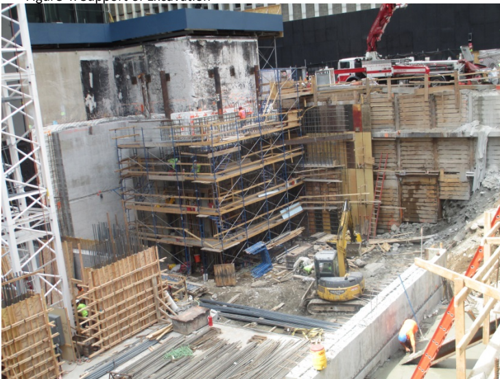
Figure 4: Support of Excavation
